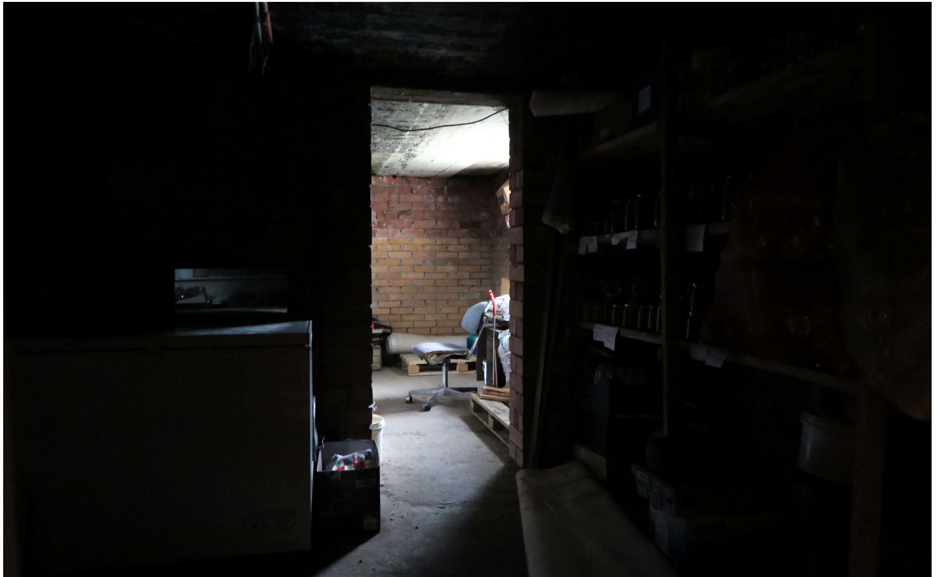
The heating room - grandfather's chair! 2024
